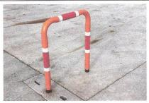
"Retro fittabe" using existing steel Sockets (above)
